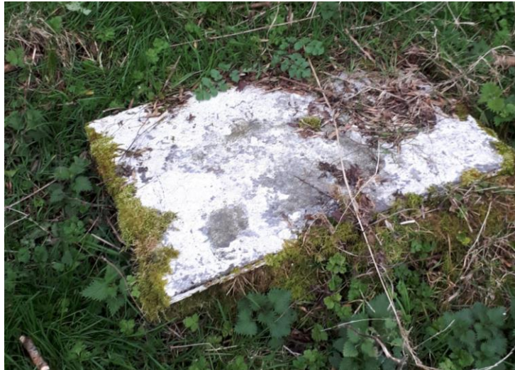
G215 _ disused borehole at Journey's End
