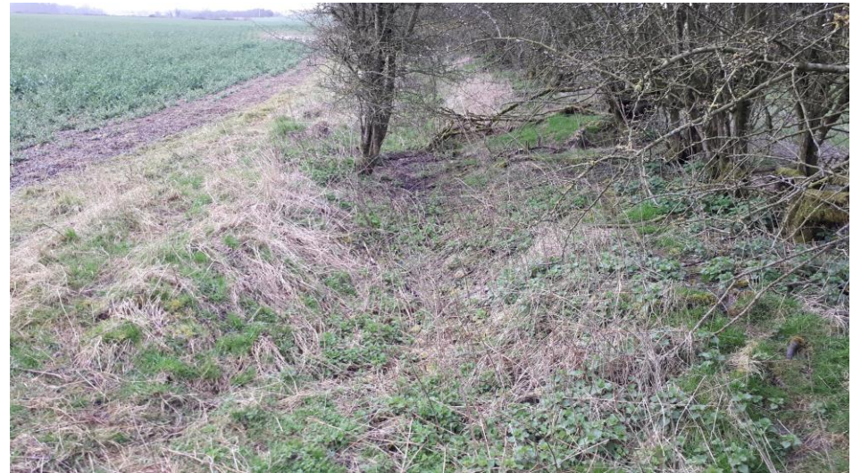
G178 _ dry road and field drain which flows to G142
