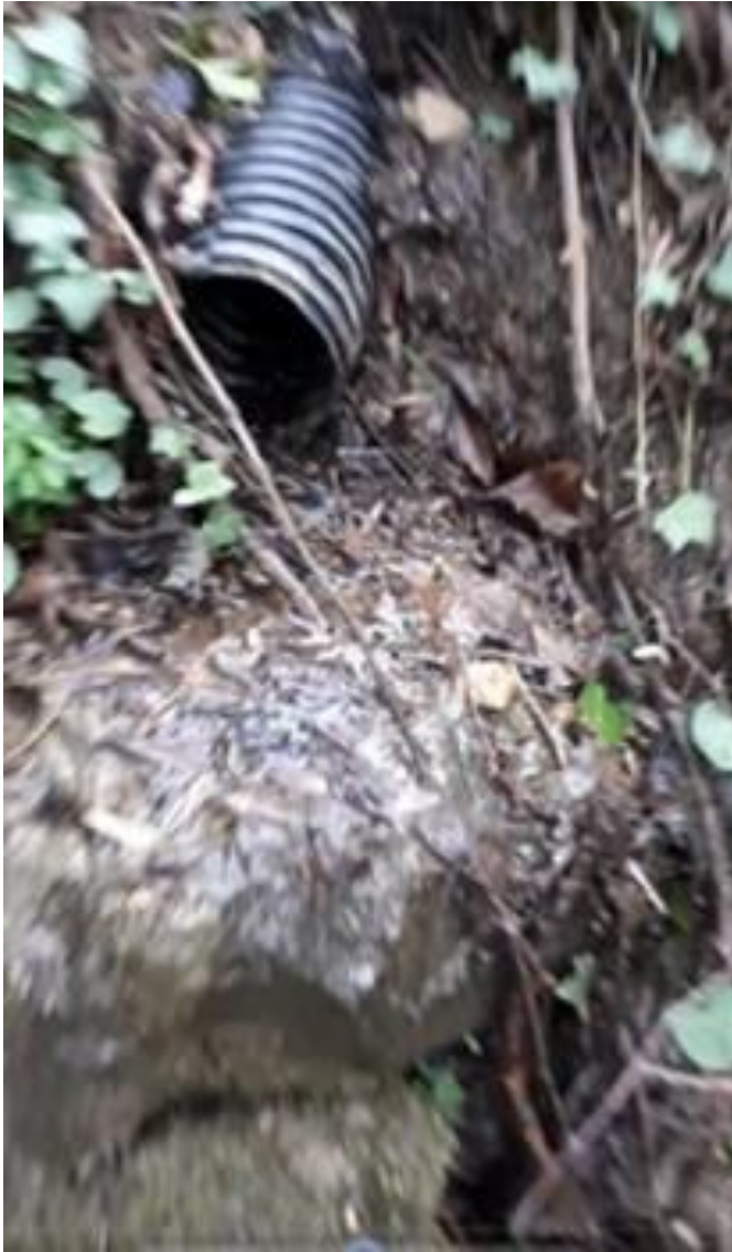
G228 _ spring flows culverted at road and flowing to drain_210319
