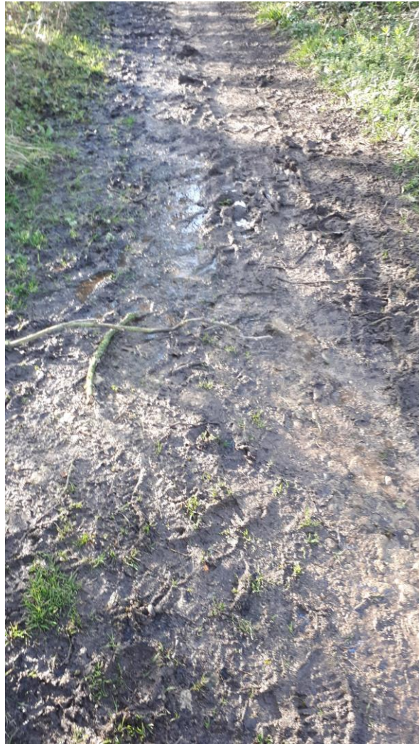
G204 _ seepage on pathway upgradient of River Churn looking W
