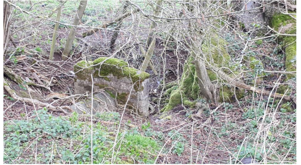
G167 _ dry spring collecter outfall at Coldwell Bottom looking NE
