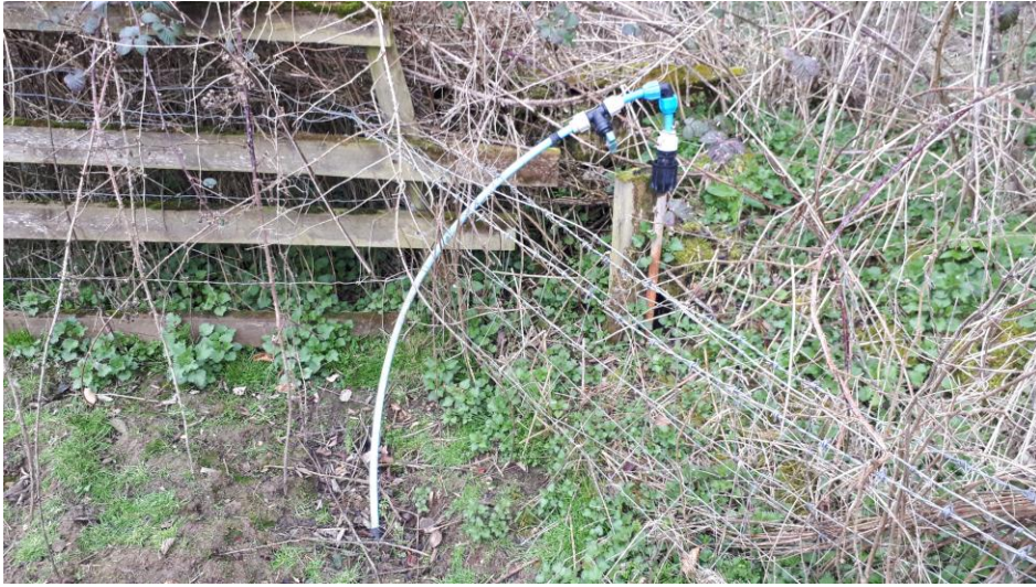
G166 _ possible abstraction point replacing old well
